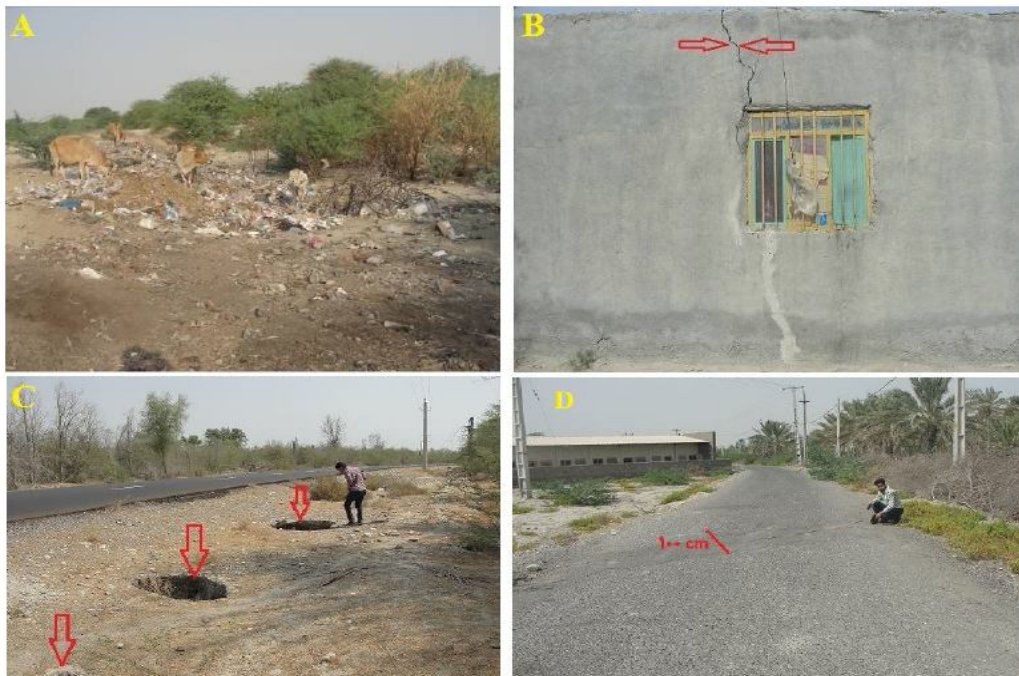
Fig. 3. The effects of the declining groundwater levels in Minab Plain. A) Drought formation, B) Crack formation in house, C) Land subsidence, D) Crack formation in road.
