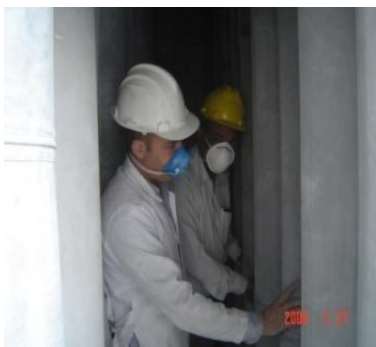
Fig.13 Step No.5-Adjusting filter bags
