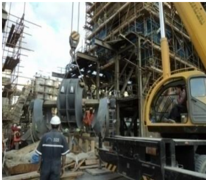
Fig.12 Step No.4-Replace old ID fan
