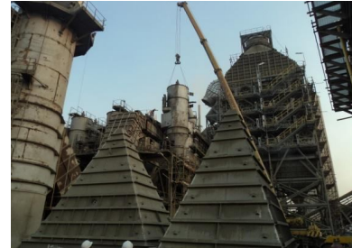
Fig.22 Demolishing of the Gravel Bed Filter
