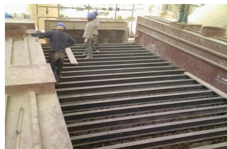
Fig.8 Step No.1-Cut the ESP roof.
