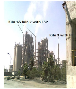
Fig.14 Comparison between ESP stacks and converted ESP into FF stack in Assiut Cement Company
