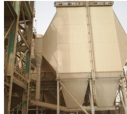
Fig.7 ESP in series – Suez plant
