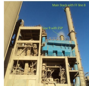
Fig.16 Comparison between ESP of line9 and converted ESP of line8 in Torah Co.
