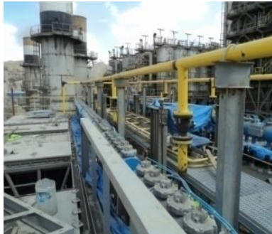
Fig.11 Step No.3-Install new gas plenum
