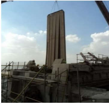
Fig.10 Collecting plates of ESP removed out.
